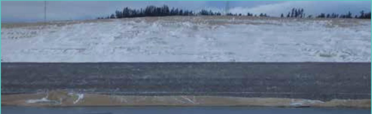
Figure 4 - Remediated Outwash Sand Slope with Rock Buttress
